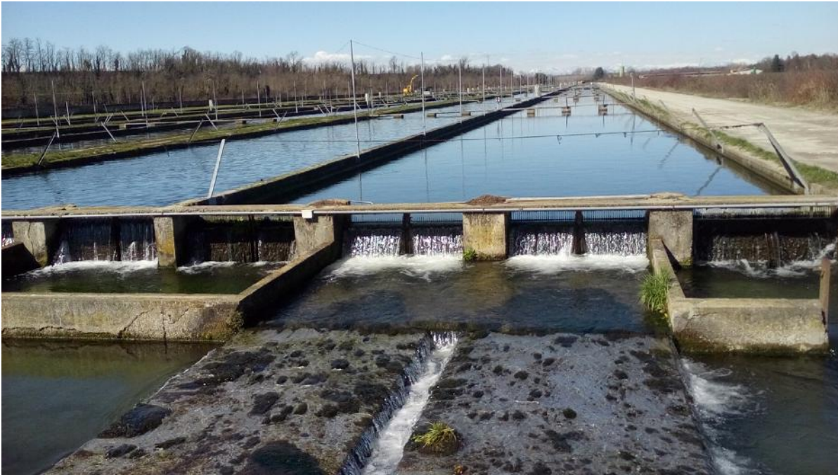
Concrete raceways
